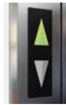
Direction arrows on entrance return
